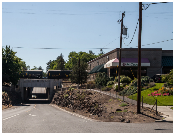
Current crossing conditions at the Franklin Avenue underpass.
